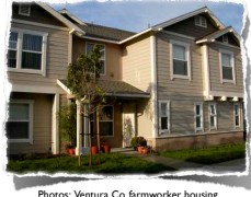
Photos: Ventura Co. farmworker housing
